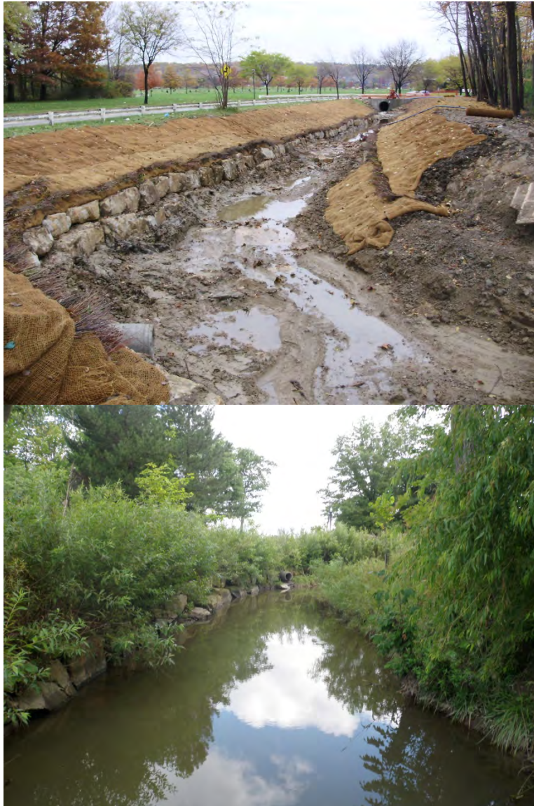
Figure 3.10. Boulder toe with live branch layering during construction and 3-years post construction (Source: Biohabitats; Oct. 23, 2011 & Aug. 14, 2014).
