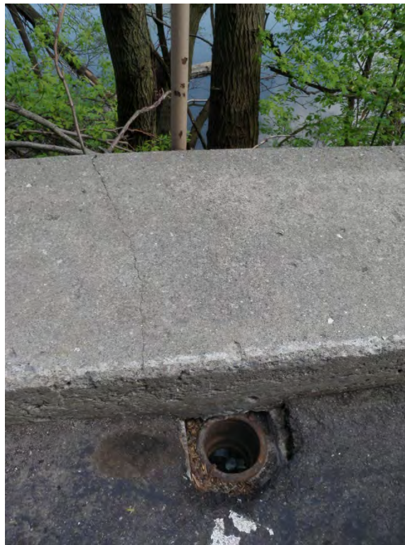
Figure 5.8. Uncovered drains at the Three Rivers Apartments (Source: Biohabitats; April 30, 2015).
